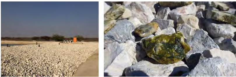
Fig. 6 Rock filter after commissioning and rock with biofilm after operational start-up.
